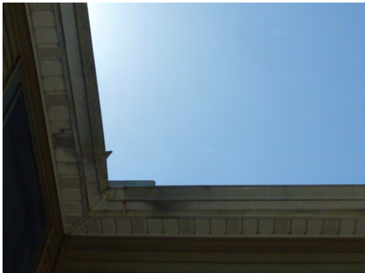
Discolored and damaged vinyl soffit and all siding is shown to be repaired through the term and replaced mid-term.
