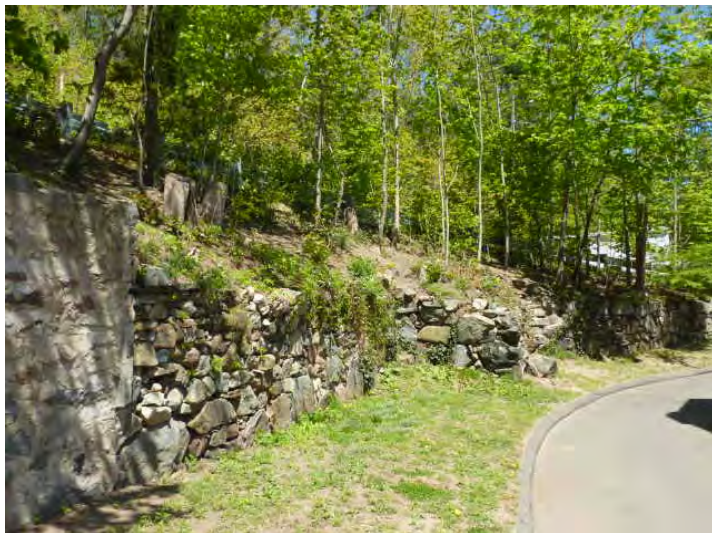
Stone retaining wall failure will continue as tree root balls behind wall continue to grow. Replacement is shown mid-term based on EUL and condition.
