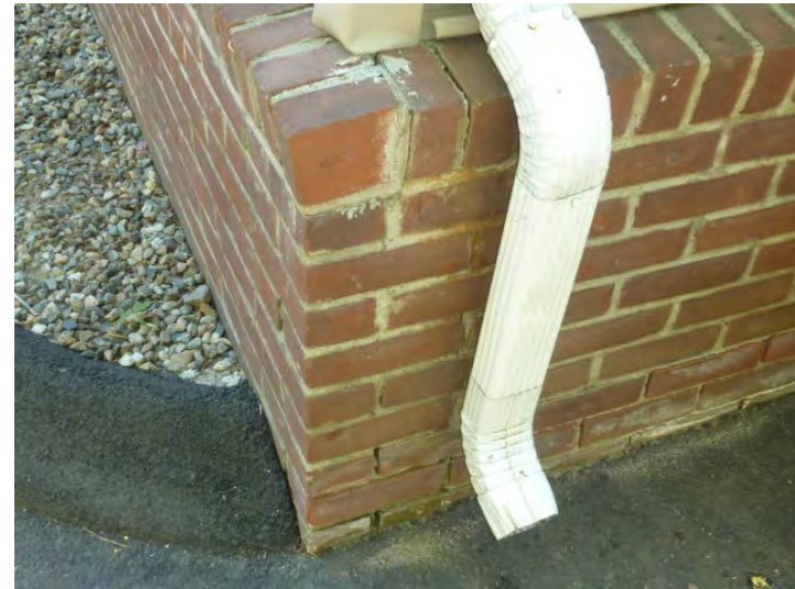
Repair and tuck-pointing of the brick water table is shown in Year 1.
