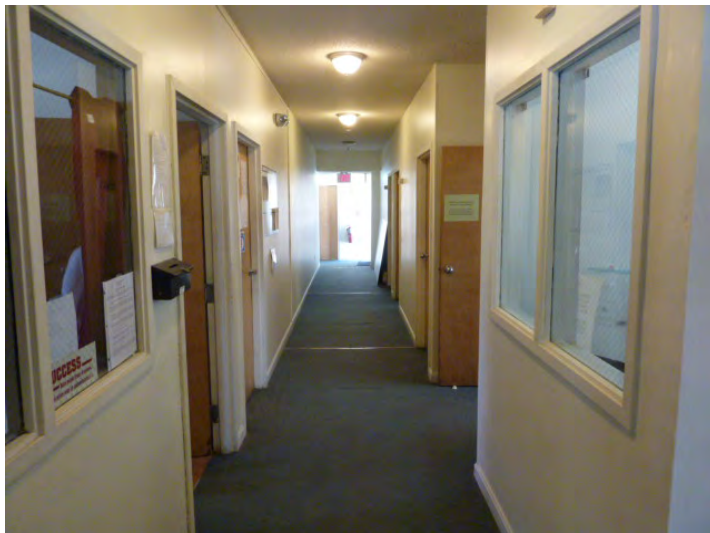
Typical first and second floor common hallway. Doors, frames and windows are not labeled with fire ratings. New fire rated doors and windows are required in Year 1.
