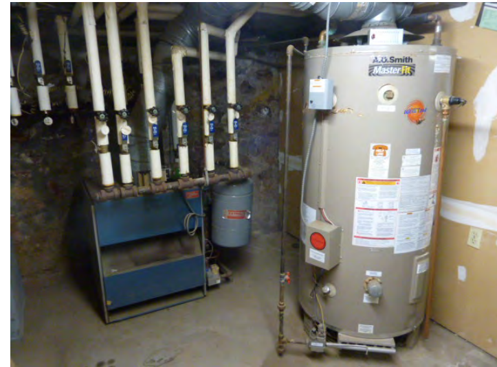
Gas-fired heating hot water boiler is original and is shown to be replaced mid-plan. Domestic hot water heater is shown to be replaced early and late.
