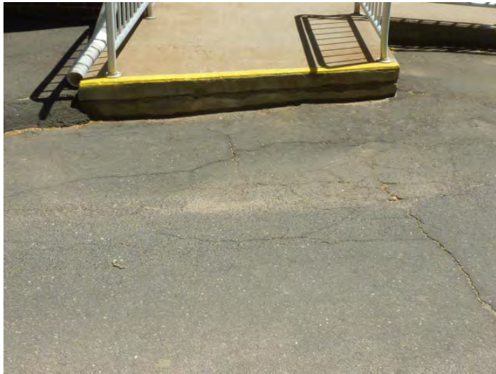
Typical cracking and sub-base failure at asphalt paving. Trip hazard is shown to be eliminated in Year 1.
