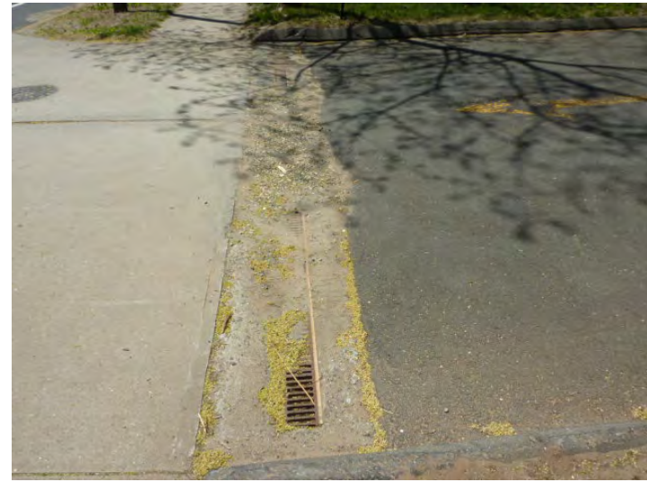
Clean and repair trench drain.
