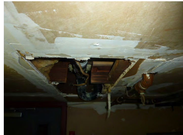
Basement ceiling is required to be a fire-rated assembly. All openings in fire rated ceilings and walls are required to be properly sealed in Year 1.
