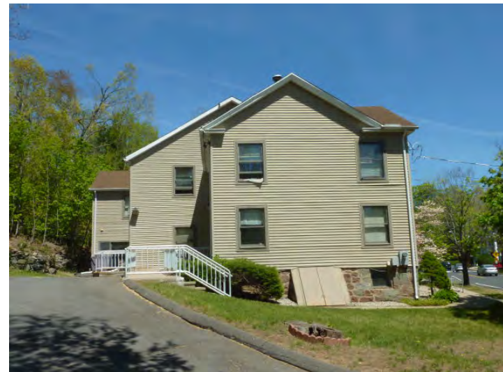
North elevation with original stone foundation wall, basement hatch door, steel pipe hand rail at stair and ramp, and several areas of buckling vinyl siding.
